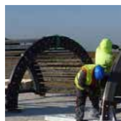
WIND TURBINE FOUNDATIONS DU GÂTINAIS WIND FARM. MONDREVILLE, FRANCE
