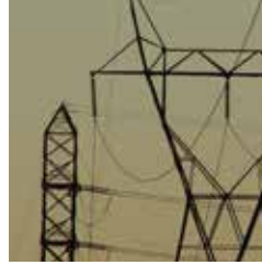
HIGH VOLTAGE DOUBLE CIRCUIT LINE CALASPARRA-ALMADENES (132 KV). MURCIA, SPAIN
