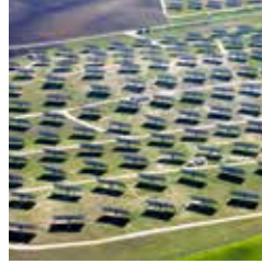
PHOTOVOLTAIC POWER STATIONS EL CORONIL (I AND II) SOLAR FARM. ANDALUSIA, SPAIN
