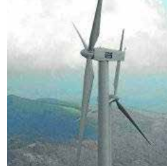
VESTAS EXPERIMENTAL WIND FARM. CANTABRIA, SPAIN
