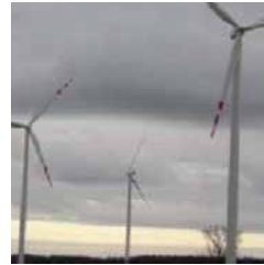
SKOCZYŁODY-SCIEKI WIND FARM IN RAWA MAZOWIECKA, POLAND
