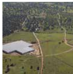
PHOTOVOLTAIC POWER STATIONS CASTILBLANCO DE LOS ARROYOS (I AND II) SOLAR GREENHOUSE. ANDALUSIA, SPAIN
