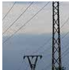
HIGH VOLTAGE LINES OF THE ROADWAY AND RAILWAY ACCESS TO THE PORT OF BARCELONA DESIGN. CATALONIA, SPAIN
